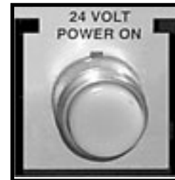
FIGURE 6-12 Power supplies operational light
